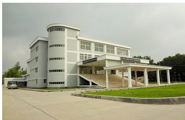
Begum Sufia Kamal Auditorium
